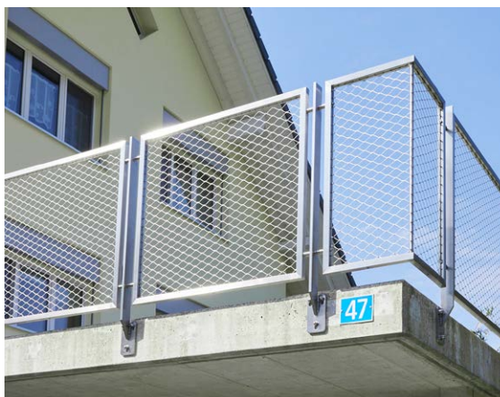
Applications of the wire rope mesh structure Webnet for railings.
